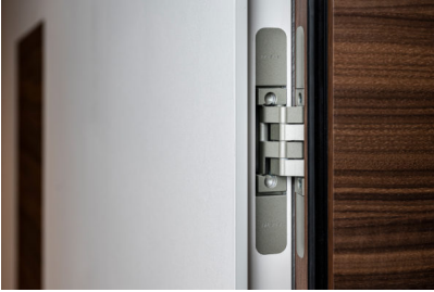
Caption 3: Clean design down to the last detail: Magnetically held cover plates hide the screws and routing areas of the hinges. Photo: Erol Gurian
