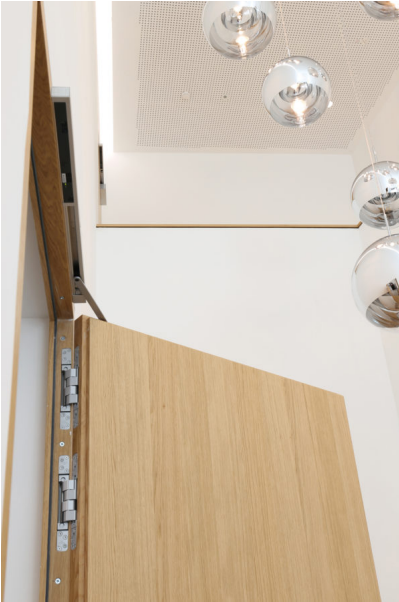
Caption 4 a - c: For oversized fire doors in the Tauberphilharmonie Weikersheim, Neuform relied on the concealed hinge "Pivota DX 300 3-D" from Basys. It has a load-bearing capacity of 300 kilograms per pair, is maintenance-free and can be adjusted three-dimensionally. Photo: Michael Meschede, Kaufungen
