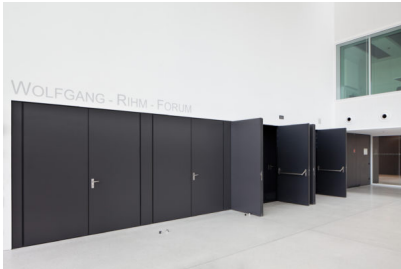
Caption 2: The fact that the door leaf and wall merge flush together is thanks to the BaSys "Pivota DX 180 3D" concealed hinge. Photo: Daniel Vieser Architekturfotografie, Karlsruhe, www.dv-a.de
