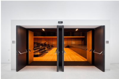
Caption 3: The heavy-duty doors by Herholz installed in the Karlsruhe multimedia complex and weighing up to 200 kilograms each, not only fulfil all the requirements for modern escape, fire and soundproof doors, they are also aesthetically flexible, thanks to the two surface finish options. The concealed BaSys "Pivota DX 180 3D" hinge supports the doors in their design and in their multifunctional application. Photo: Daniel Vieser Architekturfotografie, Karlsruhe, www.dv-a.de
