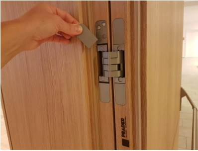
Caption 5: All of the concealed hinges installed in the "Cristal" hotel are from the designer range; here, the magnetically-held cover plate ensures a screw-free appearance. Photo: BaSys
