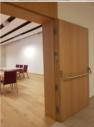
Caption 4: The special doors for the conference rooms were developed with special soundproofing requirements. Photo: BaSys
