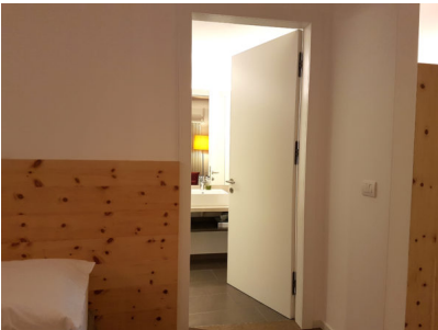
Caption 3: As with the dividing doors, the bathroom doors are fitted with the "Pivota DX38" for 60-kilogram doors. There are a total of 250 of these hinges installed throughout the "Cristal" hotel. Photo: BaSys
