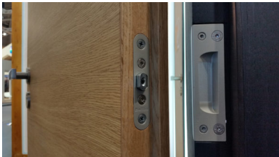
Caption 2: With the separate hinge safety mechanism, entrance doors can be secured to resistance class RC3 regardless of the type of hinge. The Basys solution is mounted on the wing side with a corresponding counterpart in the frame and remains adjustable for secure connection. Photo: Basys
